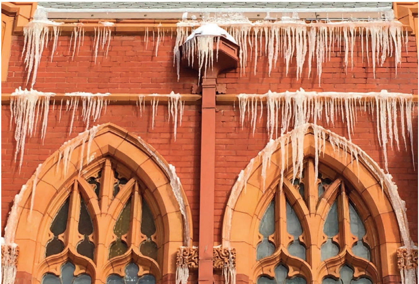
Before the gutters were fixed, the south side of the exterior of the church would be covered in ice. Photo courtesy Burt Munro.
