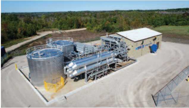
The Hydrostor facility in Goderich, Ont.
