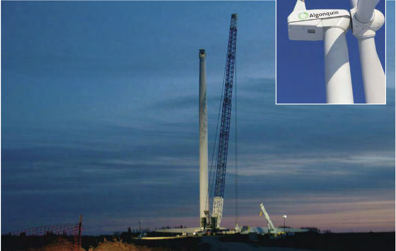
Late night construction of a Red LilyWind Project windmill. Inset: Algonquin Power Co. provides operation and supervision services to the project.
