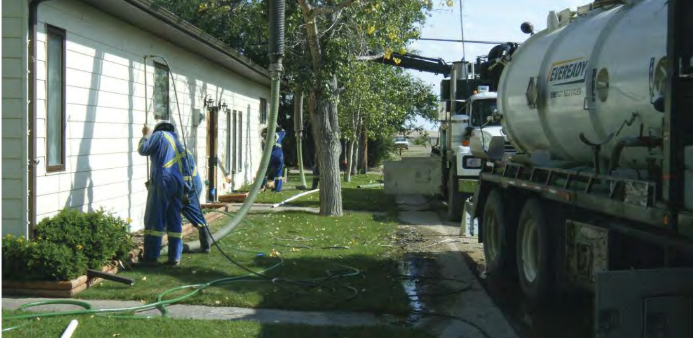
Workers installing recovery wells around a house.
