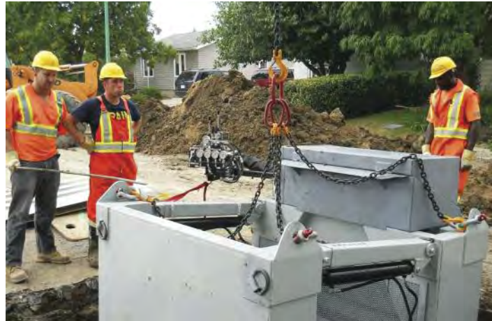
A work crew uses the Service Connector excavation cage and winch.
