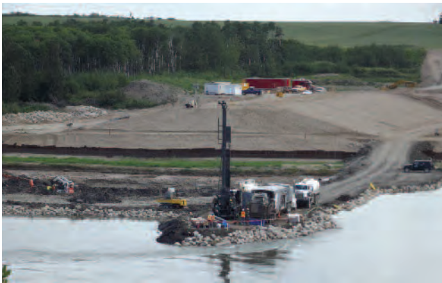
Summer pumping well installation at the site of the Ministry of Highway's St. Louis Bridge project.
