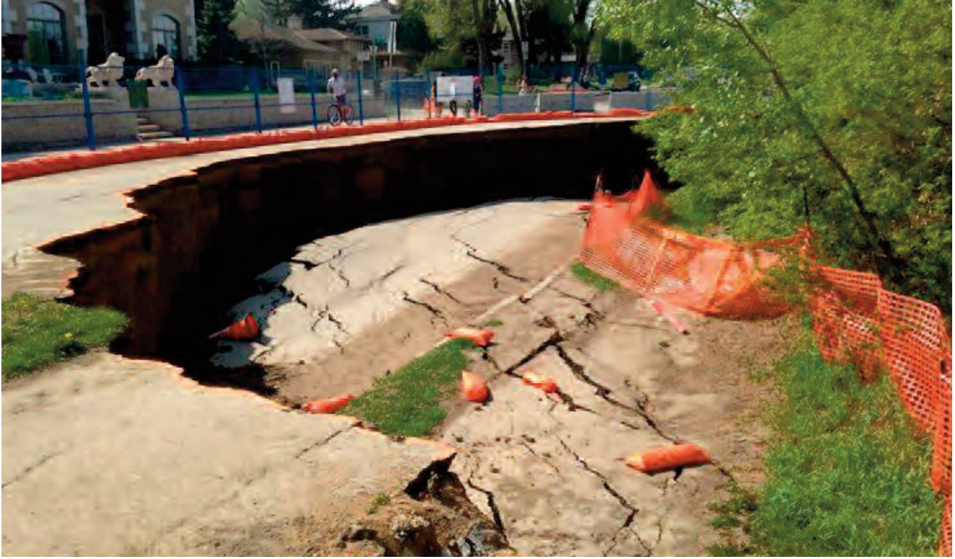
Cherry Lane Road collapse in Saskatoon
