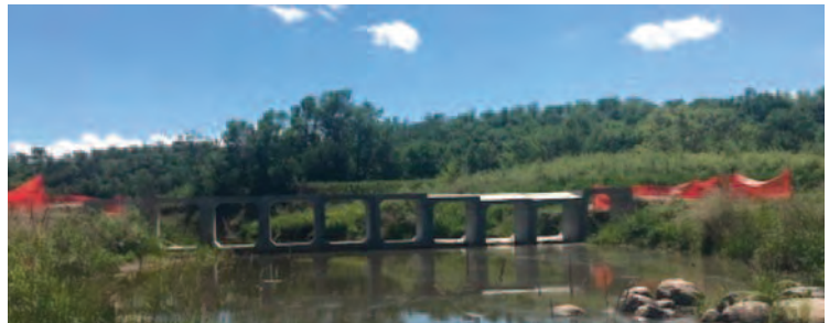
Wakamow Valley culvert bridge
