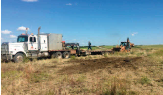
Land is returned to its original state following well reclamation.
