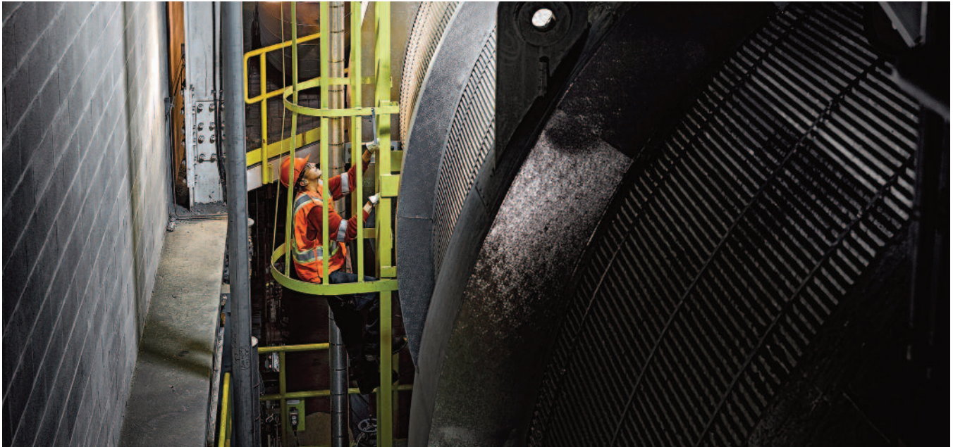
SaskPower’s Carbon Capture and Storage (CCS) facility near Estevan
