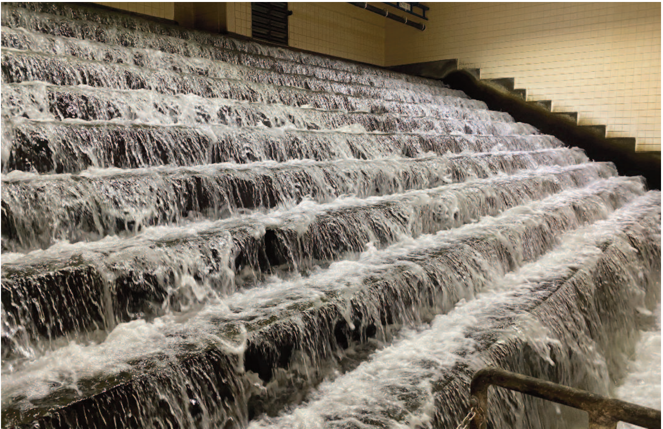
The possibility of our water supply becoming contaminated with COVID-19 is a non-issue, according to Ryan Johnson, P.Eng., general manager at Buffalo Pound Water Treatment Plant.
