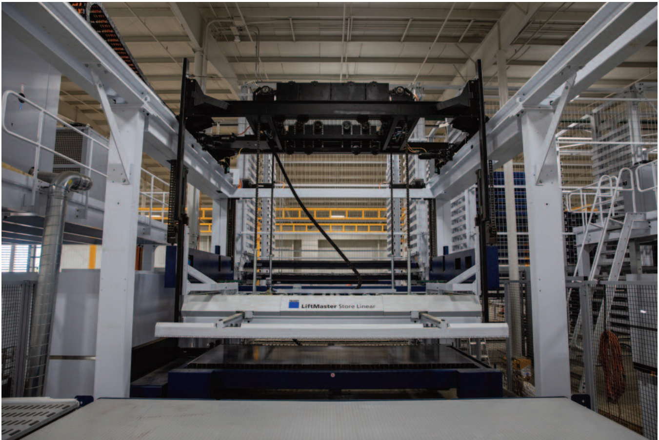
Stopa lift: The 18-tower STOPA storage system features 375 storage locations.
