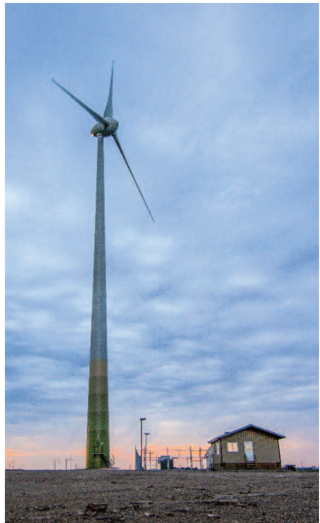
This hybrid facility came online in 2013 as a partnership between Cowessess First Nation and Saskatchewan Research Council.
