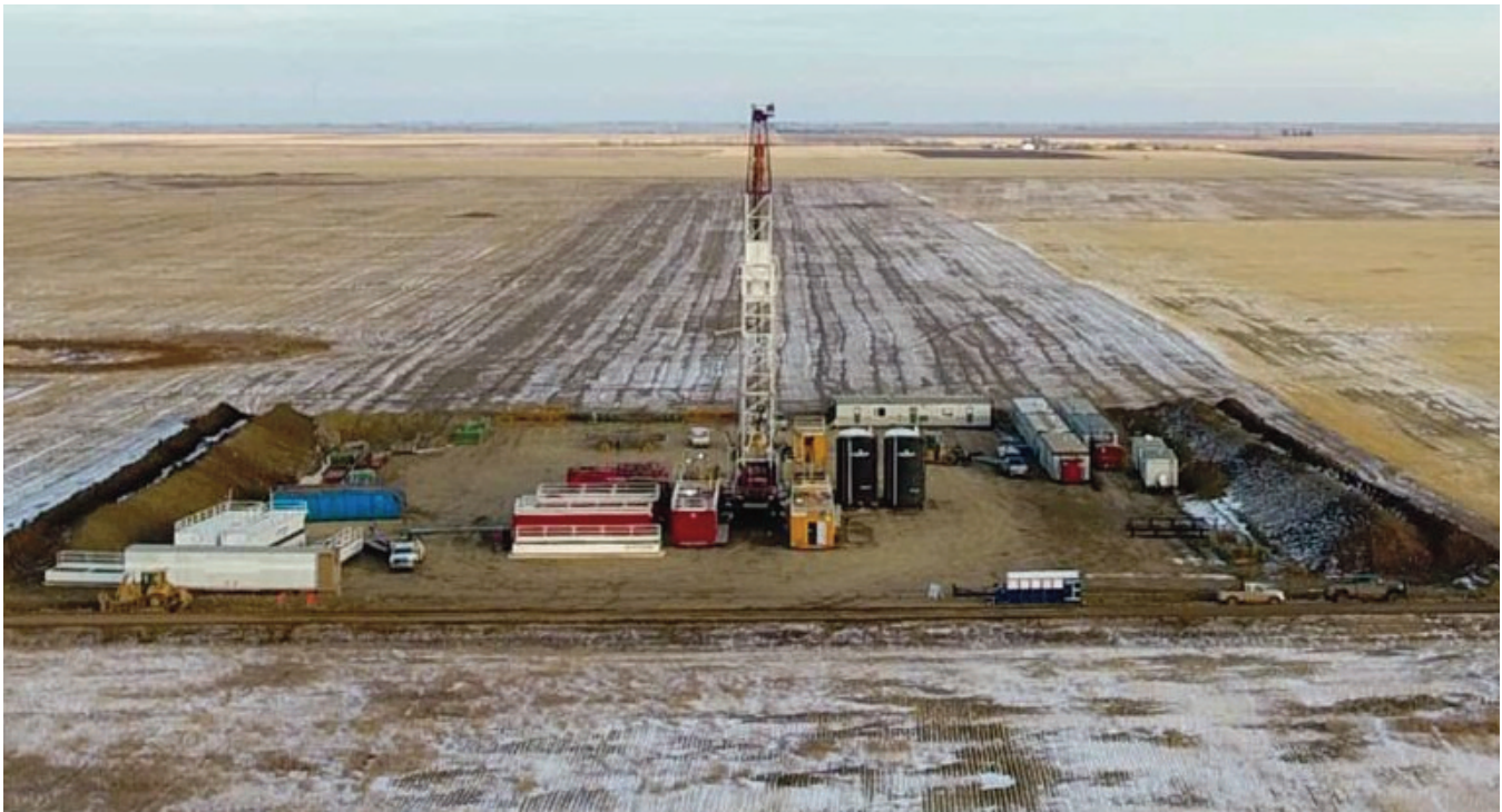
DEEP drilling rig on site of geothermal project.
